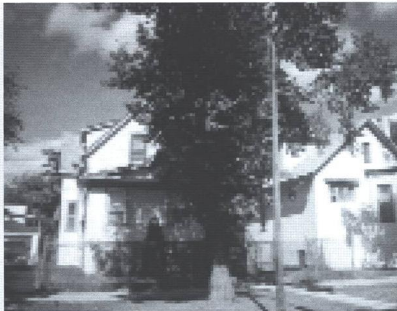
Shown above is one of the homes that landlord Deborah Mitchell cares for in Chicago's Austin neighborhood.
